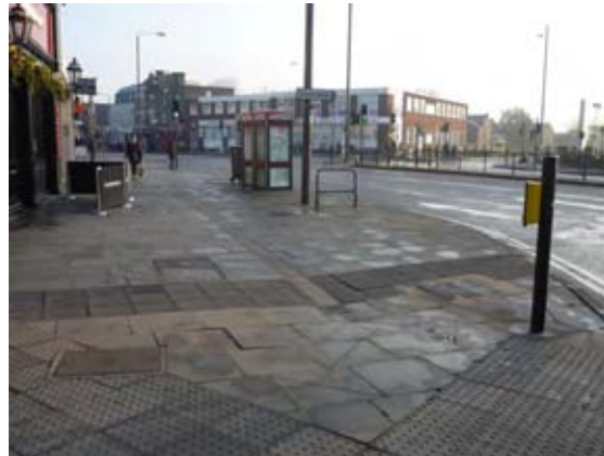
(Left) Raised delineator and tramline paving indicate the beginning of a cycle track on a partially separated footway. The symbol in the foreground shows a shared area. (Right) Corduroy paving is used to bound a shared area at a crossing, with footway for pedestrians only beyond this.
