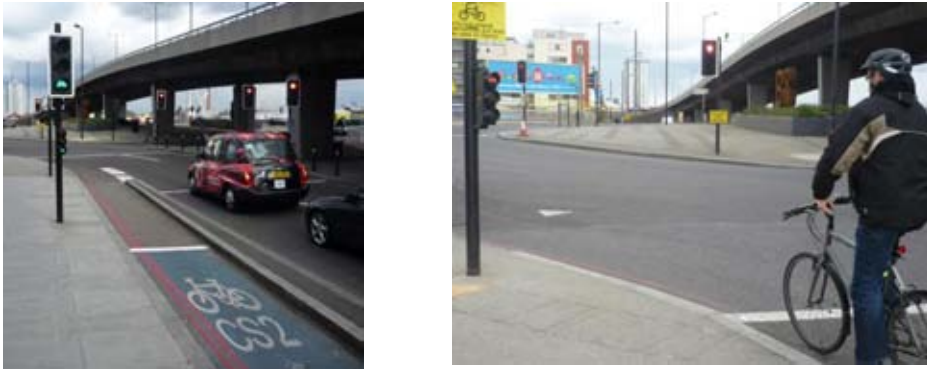
Cycle gate at Bow: (left) segregated approach and first cycle stop line, and (right) advanced cycle stop line. Trial low-level cycle signals (used as repeaters) are mounted below the main signal heads.
