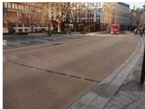
Wide crossing, consisting of two parallel stand-alone, signal-controlled crossings, with contrasting surface treatment, St Paul's Churchyard, City of London
