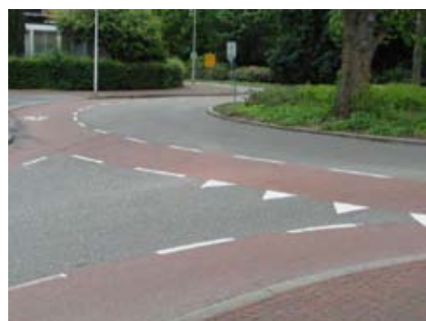
Roundabout with annular cycle lane in Utrecht (sharks' teeth markings mean 'give way')
