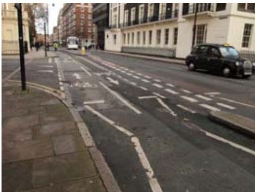
Difficulties in highlighting to all road users that a two-way cycle track is crossing a side road – Tavistock Place, Camden (left) and CS3, Cable Street (right). There is no standardised combination of road marking for this, so efforts are made on a site-by-site basis to demonstrate the intended priority.
