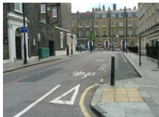
Footway build out on street with contraflow cycling
