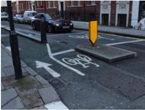
Two-way facilities can lead to awkward transitions when joining with one-way provision (left) Consideration needs to be avoiding pinch-points at bends where effective width is squeezed (right)
