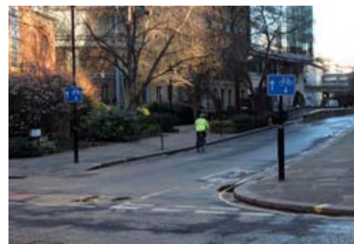
Contraflow cycling in City of London using the diagram 960.2 sign: advisory contraflow at Aldermanbury Street (left) and at Noble Street (right) using advisory lane markings only at the junction
