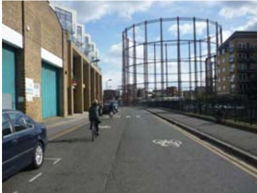
Gaps between speed cushions are in line for cyclists, reinforced by cycle symbol positioning
