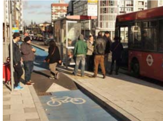
Bus stop bypass at Stratford High Street, showing pedestrian crossing over cycle track in detail
