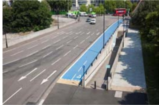
General traffic lane converted to off-carriageway tracks at Wandsworth Gyratory
