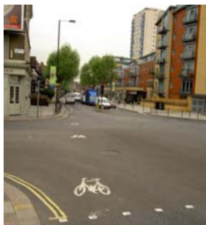
Well-placed cycle symbols through a junction to show a recommended route for ahead cyclists (left). Poorly placed cycle symbol on a bend (right).
