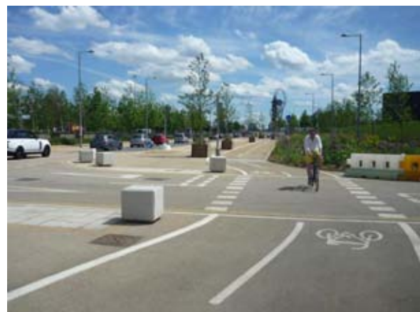
Bent-out cycle tracks with unambiguous priority over a side road junction at Waterden Road, Hackney. In this instance, the bending is less apparent because the tracks are already set well back from the carriageway.
