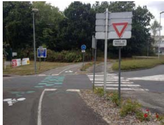
Off-carriageway cycling at roundabout in Nantes – motorists give way to crossing cyclists
