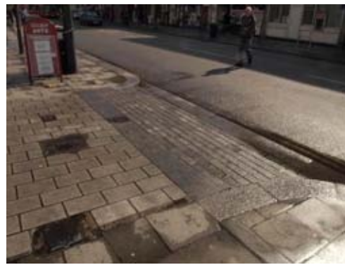
Block-paved entry treatment with tight corner radii – Walworth Road, Southwark
