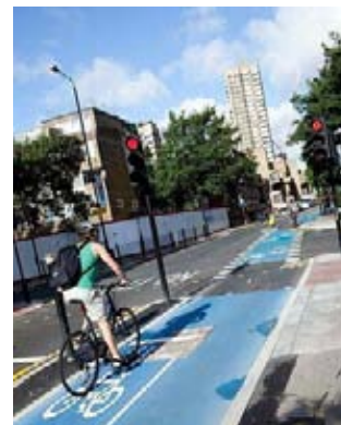
Difficulties in highlighting to all road users that a two-way cycle track is crossing a side road – Tavistock Place, Camden (left) and CS3, Cable Street (right). There is no standardised combination of road marking for this, so efforts are made on a site-by-site basis to demonstrate the intended priority.
