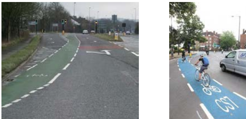
Use of dashed lane markings and surface colour to highlight a cycle lane to motorists seeking to enter a left-turn lane
