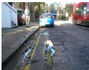
Standing water due to uneven or slack gradients, blocked gullies, rutting of surface or leaking water valves.
