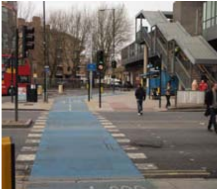
Type [1]: parallel crossings at Westferry and West India Dock Road. Ladder and tramline tactile paving are used for transition from track to shared area.
