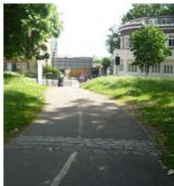
Use of granite setts to slow cyclists through parks and, right, at a courtesy pedestrian crossing
