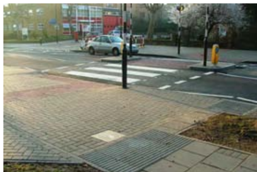
Conventional zebra crossing (left), with buff blister tactiles. Shared area on either side of the zebra (right) to legitimise cycle use of the crossing.
