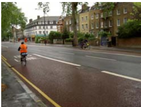
With-flow bus lane (left) and contraflow lane with 'bus and cycle' marking (right)
