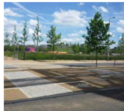
Use of granite setts to slow cyclists through parks and, right, at a courtesy pedestrian crossing
