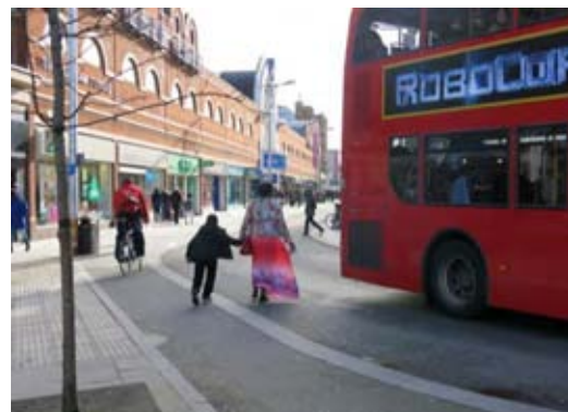
Contraflow cycle track at footway level in London – distinction with cycleway is less clear
