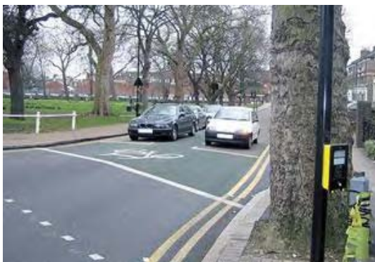
Central lead-in at signalised junction (left). Long central lead-in to allow for left-turn flare, positioned to facilitate overtaking stopped buses (right).
