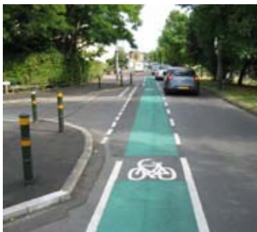
Buffer between lane and give way markings, and use of colour
