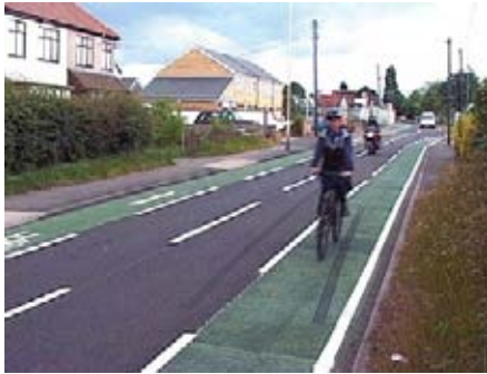
Advisory lanes used for a visible cycling facility where carriageway width is limited
