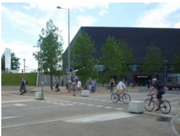
Bent-out cycle tracks with unambiguous priority over a side road junction at Waterden Road, Hackney. In this instance, the bending is less apparent because the tracks are already set well back from the carriageway.
