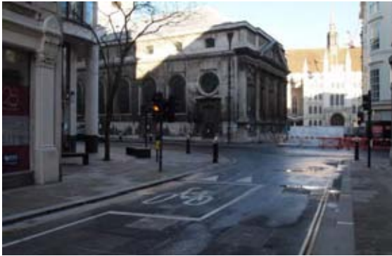
Narrow lead-in lane on street with no centre line, so vehicles tend not to queue over the lead-in lane
