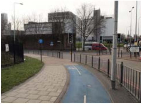
Toucan crossings are often used to carry off-carriageway tracks through or around junctions
