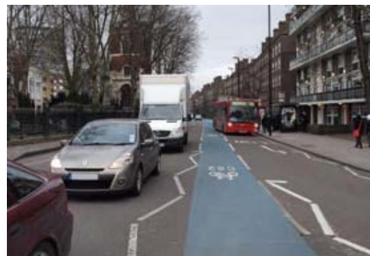
Central lead-in at signalised junction (left). Long central lead-in to allow for left-turn flare, positioned to facilitate overtaking stopped buses (right).
