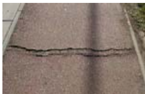
Surface cracking or excessive rutting
