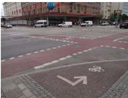
Two-stage left-turn marking at junction in Stockholm (left); and cyclists in different streams in Copenhagen (right) – left turners are heading to the waiting area to the right
