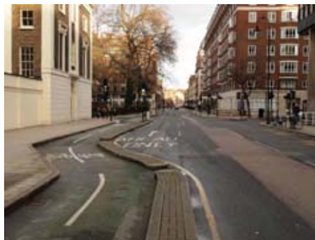
Track at Tavistock Street, Camden, forming a parallel carriageway and simplifying movement through a four-arm junction (but note the need for the left-turn ban).
