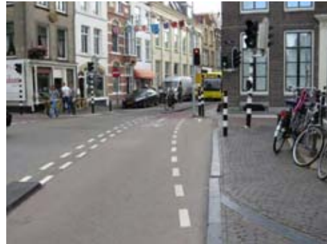
Cyclists using the crossing to turn left are directed to wait on the right, allowing others to continue ahead unhindered
