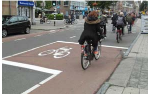
ASLs with lead-in lanes are also used in other countries – as in this example from Utrecht
