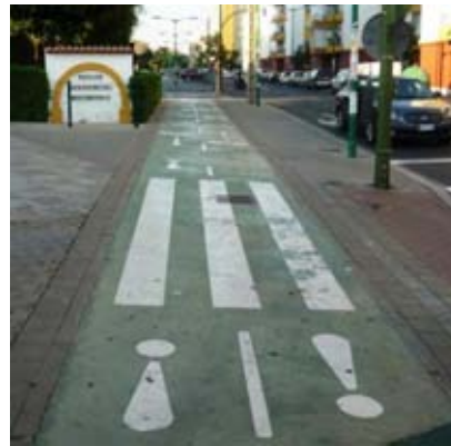
Pedestrian crossing over a cycle track in Seville, with extra warning for cyclists
