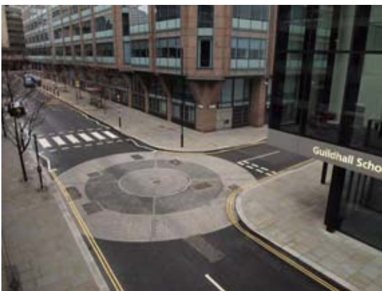
Informal roundabouts at Moor Lane, City of London (left) and Bexleyheath town centre (right), both of which have a 'roundabout-like' feature in the carriageway
