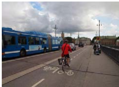
Segregated lanes/tracks with low kerb upstands – in Utrecht (left) and Stockholm (right)
