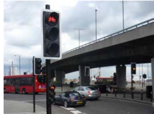
High-level red cycle aspect (with low-level cycle signal used as repeater) at Bow roundabout
