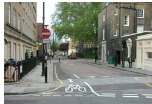
No entry with 'except cycles' plates, and raised table entry
