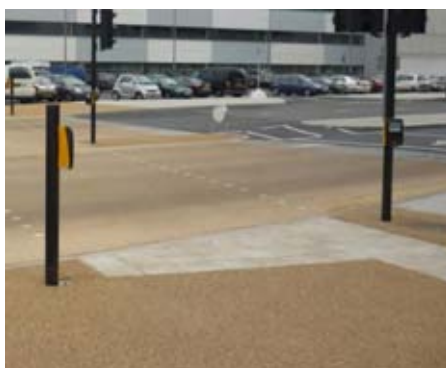
Red and grey blister tactile paving used at crossings
