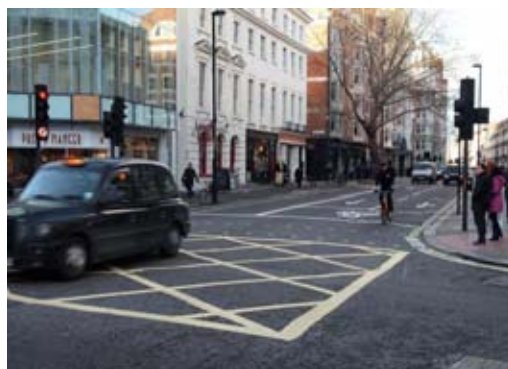
ASL across two lanes only from one-way street (offside lane is a bus lane) – Gower Street, Camden
