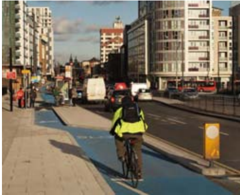
Bus stop bypass at Stratford High Street, showing pedestrian crossing over cycle track in detail
