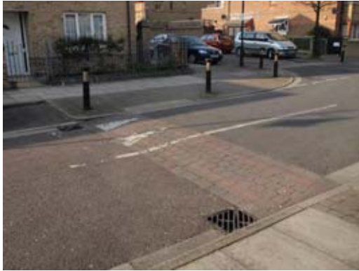
Sinusoidal ramp in block paving
