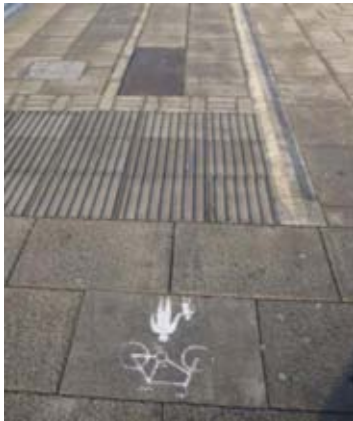
(Left) Raised delineator and tramline paving indicate the beginning of a cycle track on a partially separated footway. The symbol in the foreground shows a shared area. (Right) Corduroy paving is used to bound a shared area at a crossing, with footway for pedestrians only beyond this.
