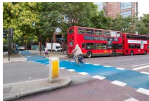
Signal-controlled cycle crossings, using elephant's footprint markings through the junction
