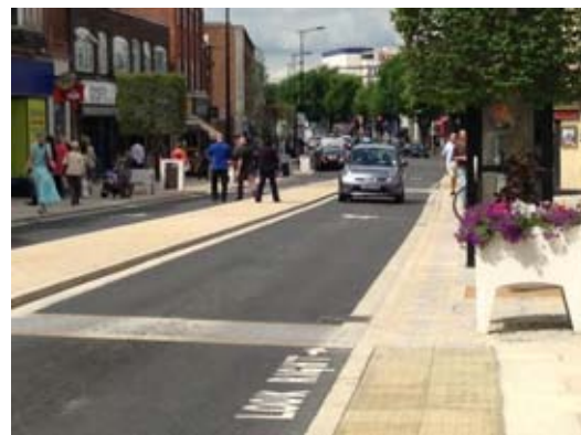
Median strip used for visual narrowing and to enable informal crossing – Hornchurch
