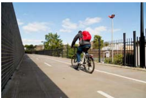
Separation on an off-highway route with few pedestrians. The high wall reduces effective width, and the cyclist is cycling on the 'wrong' side.
