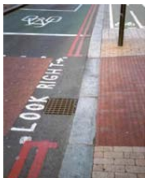
Red and grey blister tactile paving used at crossings
