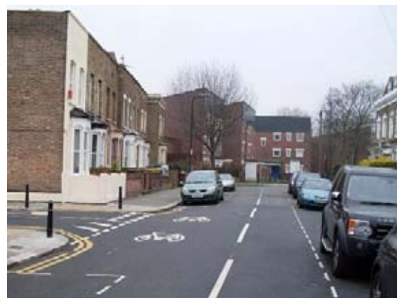
TSRGD diagram 1057 symbols positioned so as to mark a cycle route through a junction
